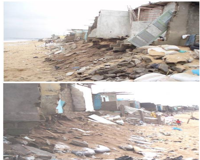
Fig. 3: Destruction of dwellings in the commune of Port Bouet (Abidjan)
